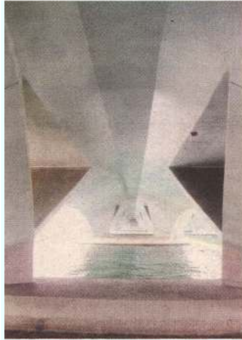
Under the Esplanade Bridge in Merlion Park
